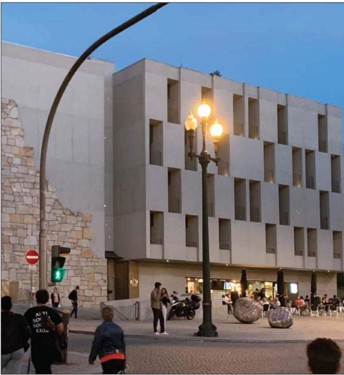
Sympathetic adaptive re-use in Oporto: retaining the façade facing the UNESCO World Heritage San Bento (St Benedict) railway station and integrating 21stC new build to re-purpose the site
