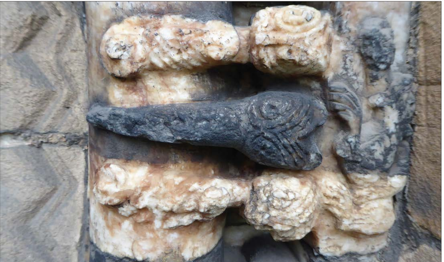
Alabaster stones at St Mary's Tutbury, showing the before and after effect of laser cleaning
