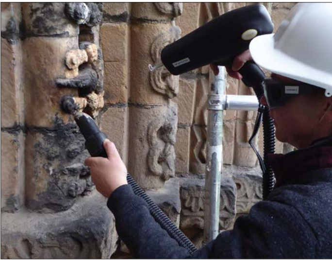
Senior Stone & Wall Paintings Conservator Sabina van de Bruck ACR laser cleaning the exterior alabaster archivolt at St Mary's Church, Tutbury
