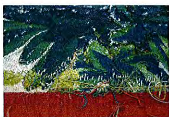
Areas of reweaving joining a patch from one tapestry into the field of another. Adhesive remains left from previously patched areas can also be seen.
