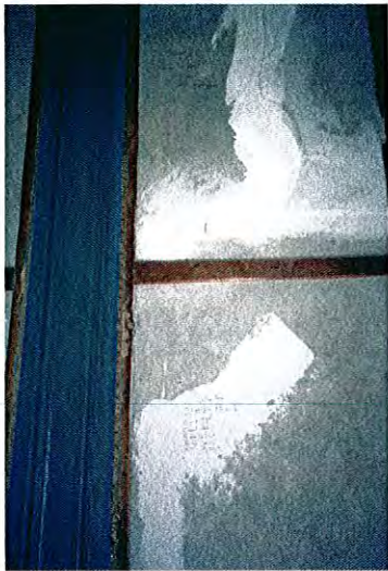
Fig 1: The wooden support frame on which the tapestries were originally nailed. The nails are still in place. Above centre are the signature of the builders of 1887. Below are those of builders who repaired the wall plaster in 1996.
