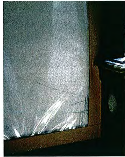
Fig. 2: A wall panel lined with polyester film and edged with a cotton twill band in preparation for the mounting of a tapestry.
