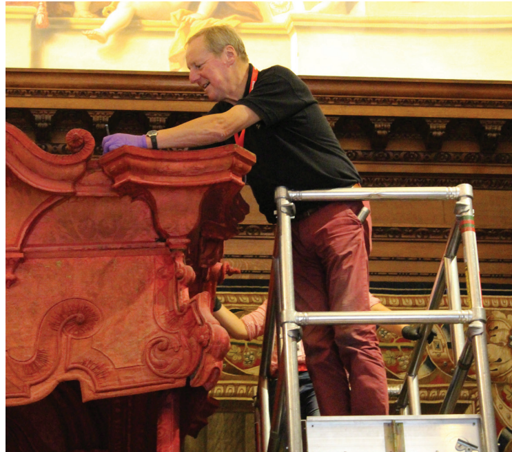
Fig. 2 Tankerdale Ltd. preparing to take down a corbel.
