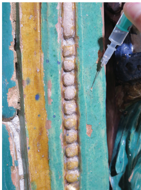
Figure 5. Injection of 10 percent PARALOID B-72 consolidant into hollow sections under the glazed surface
