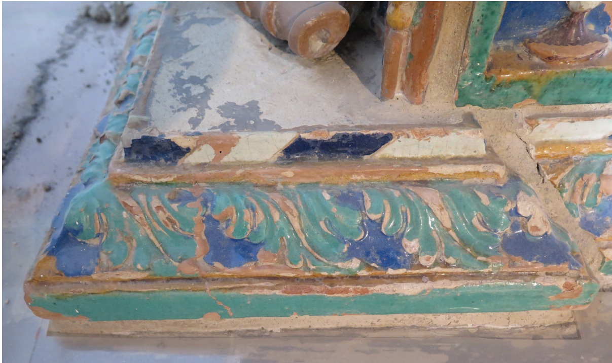
Figure 2. Detail of a corner tile from the top level before intervention, showing losses of glaze, paint drips, plaster of Paris fills, and overfilled grouts
