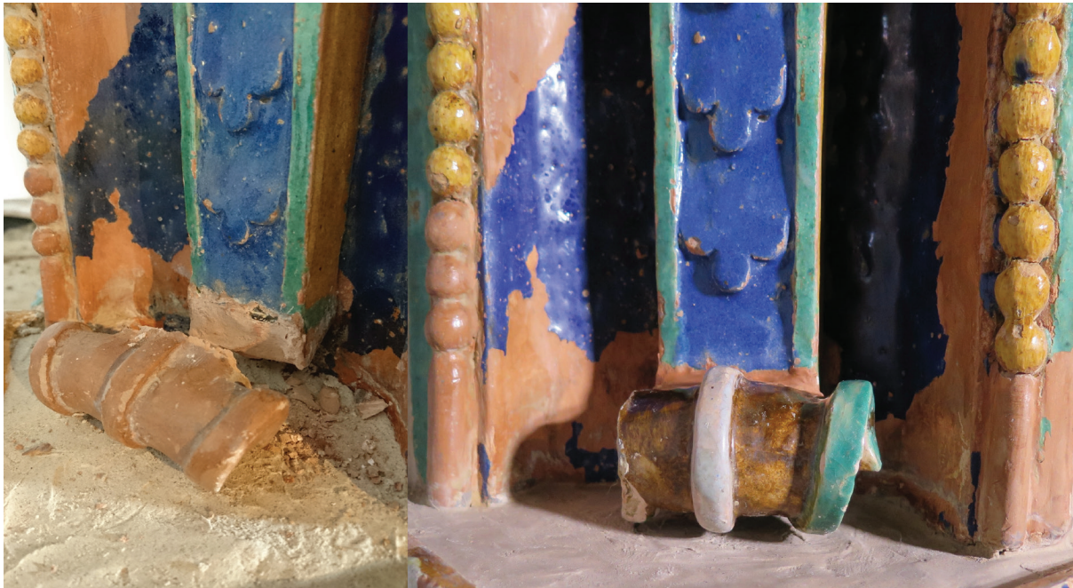
Figure 8. Detail of the replica of the section found in the archive (left), and the original fragment reinstated (right)
