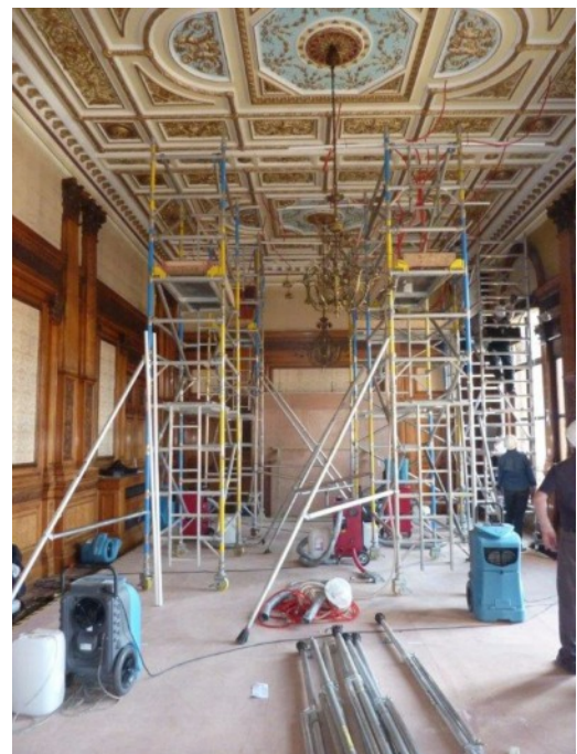
Figure 1 Satinwood Suite, a few days after the flood. The most badly affected area was the south/west corner and heading left beyond fireplace at the back of this picture. The alabaster fireplace was boxed up for protection and the heavy plaster ceiling re-pinned to prevent collapse.
